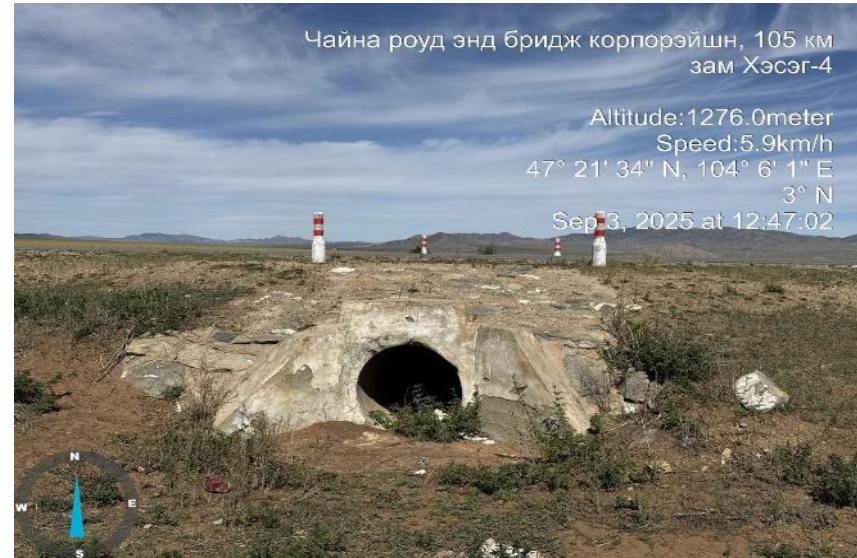
Figure 1. Current condition of drainage culvert, Section 4
