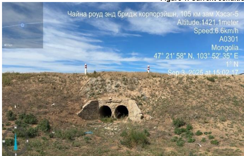
Figure 2. Current condition of drainage culvert, Section 5
