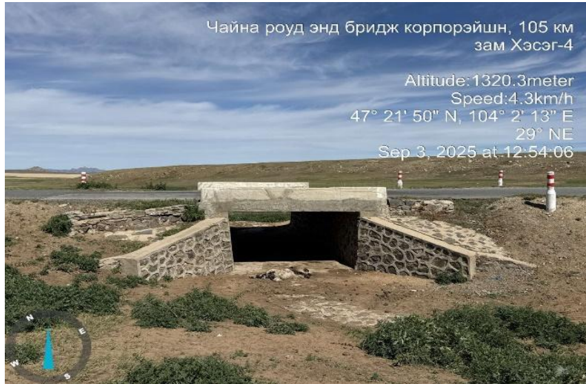
Figure 1. Current condition of drainage culvert, Section 4
