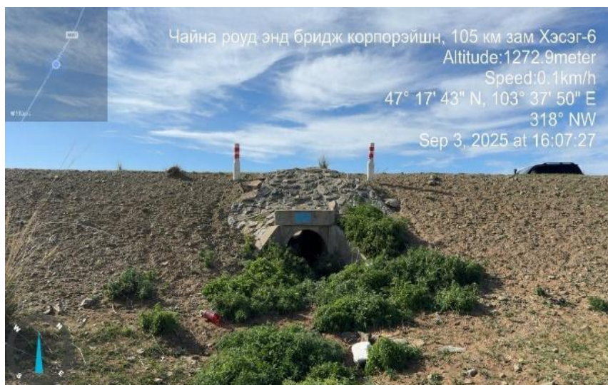
Figure 3. Current condition of drainage culvert, Section 6
